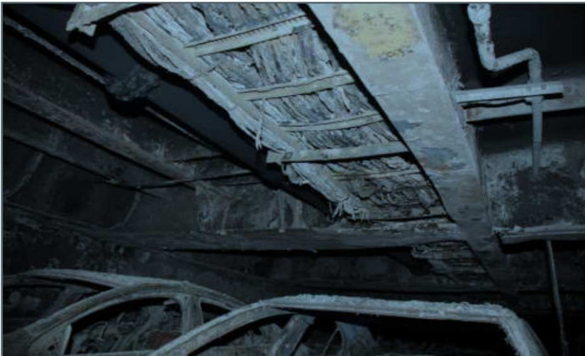
Figure 54: Destroyed cable routing and deformed girders beneath the ceiling
